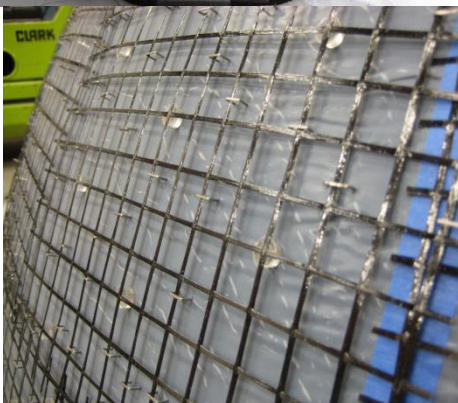
Figure 5. Foundation ring poured, using forms set on right, with tie-in fiberglass mesh embedded in ring. Twelve "orange peel" spherical segments are now bolted together, with a shim in each joint, to allow easy release of form segments from cured thin-shell-concrete dome. The gray surface is Teflon, for easy form segment release from cured concrete. Ready for installation of "tiled" C-Grid sections, with SS staples captured in 60 mil rubber layer under the Teflon: Figure 4. Proof-of-concept prototype is 2.8 m equatorial diam, 5/8 sphere vol. This project will scale-up to 6-7 m diam via tooling on which to build larger "orange peel" and top cap fiberglass forms panels, as shown.
