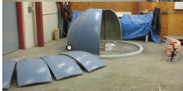
Figure 5. Foundation ring poured, using forms set on right, with tie-in fiberglass mesh embedded in ring. Twelve "orange peel" spherical segments are now bolted together, with a shim in each joint, to allow easy release of form segments from cured thin-shell-concrete dome. The gray surface is Teflon, for easy form segment release from cured concrete. Ready for installation of "tiled" C-Grid sections, with SS staples captured in 60 mil rubber layer under the Teflon: Figure 4. Proof-of-concept prototype is 2.8 m equatorial diam, 5/8 sphere vol. This project will scale-up to 6-7 m diam via tooling on which to build larger "orange peel" and top cap fiberglass forms panels, as shown.
