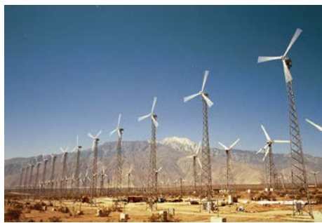
Figure 2. SEIG mode test on one of AASI's 13 Palm Springs 50 kW wind turbines, variable speed, "wild AC" to "wild DC" to resistive load. Self-excitation lost at low windspeed. No grid connection. https://vimeo.com/160472532
