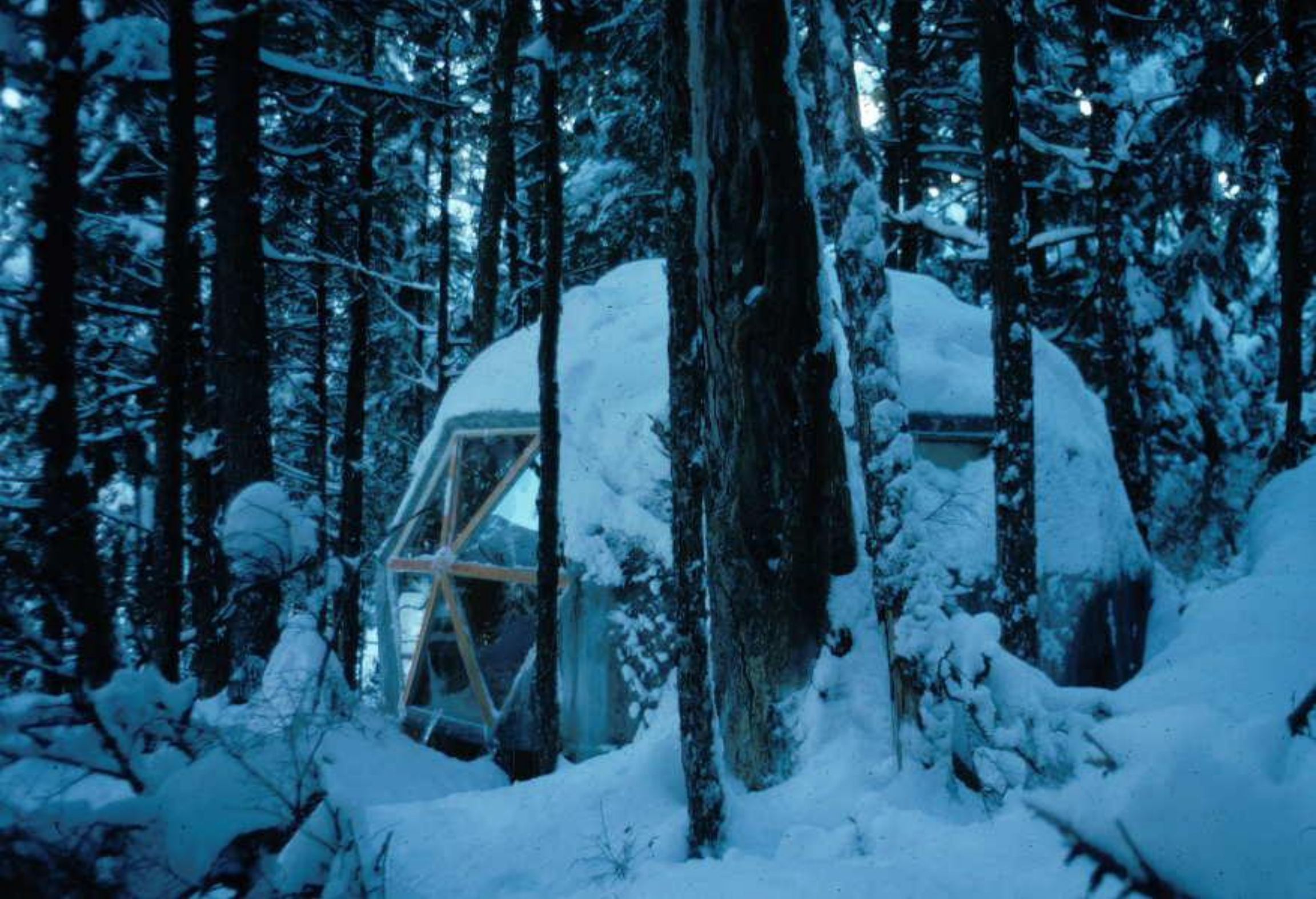
Juneau, AK 1974: 16' diameter concrete dome: \frac{1}{2} " thick, \sim \frac{5}{8} sphere 3
